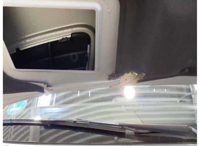
Damage 1: Bonnet: Insulation lining - Damaged - Replace
