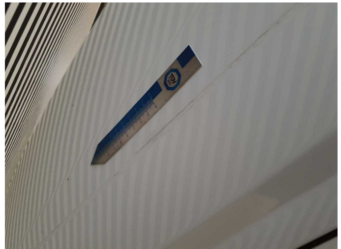
Damage 7: Roof: Roof rail - left side - Dent / paintcoat damage - Paint
