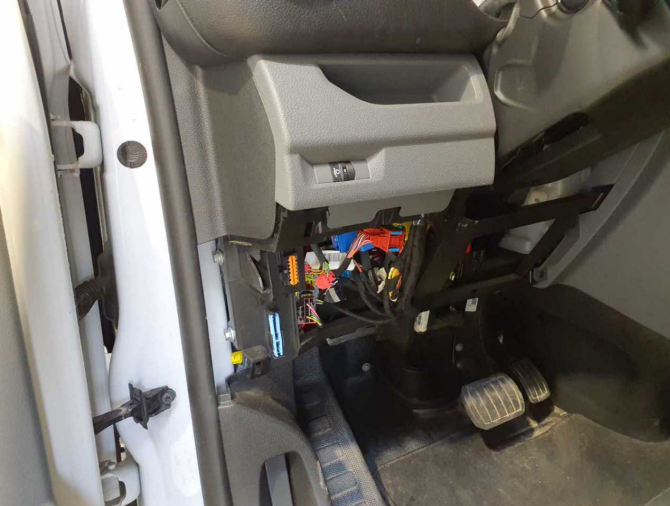
Damage 4: Electronic systems: Electronic systems - Specify findings - Perform diagnosis
