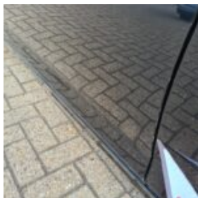
Damage Type Door-edge chipped
