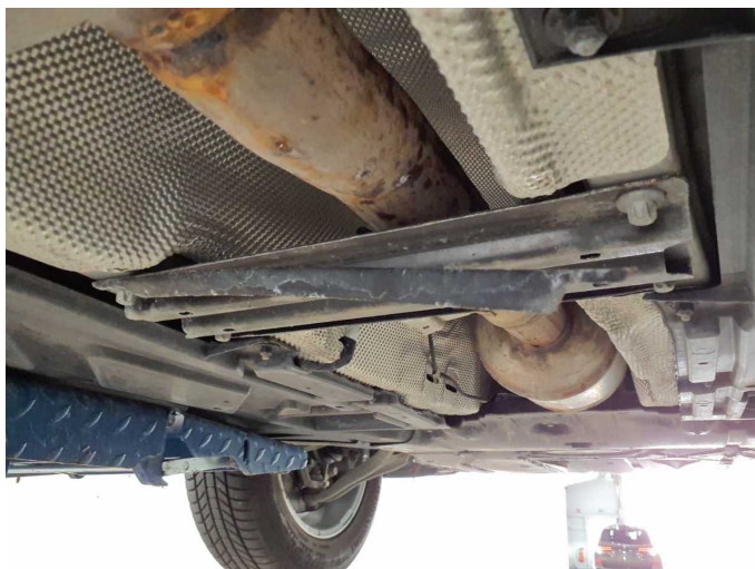
Damage 8: Body: Underbody - Broken / torn - Replace
