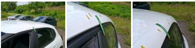
Roof pillar L, Hail damage, Repair and paint (complete)
