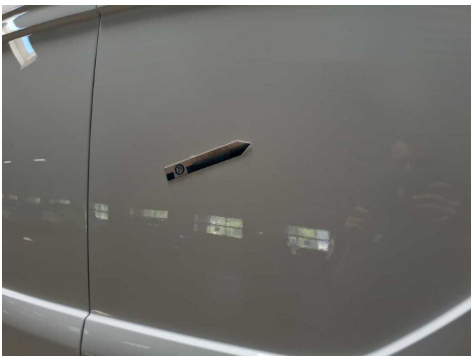
Damage 4: Boot lid / rear door: Rear door - right side (l) - Dent / paintcoat damage - Repair and paint
