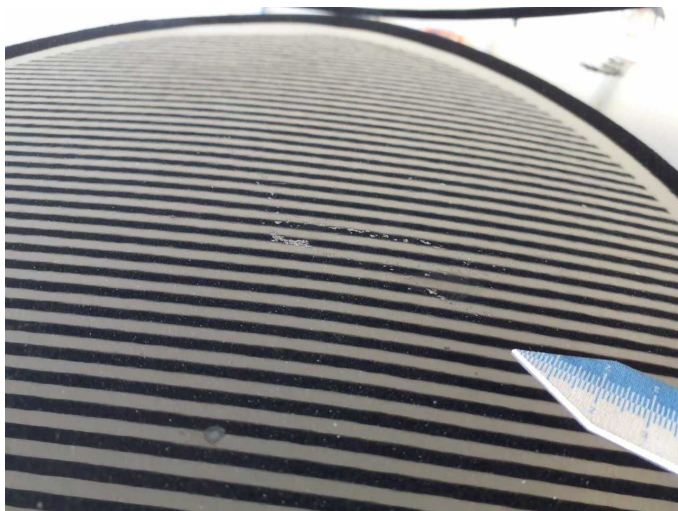
Damage 21: Roof: Roof (Anätzung) - Paint defect - Repair and paint
