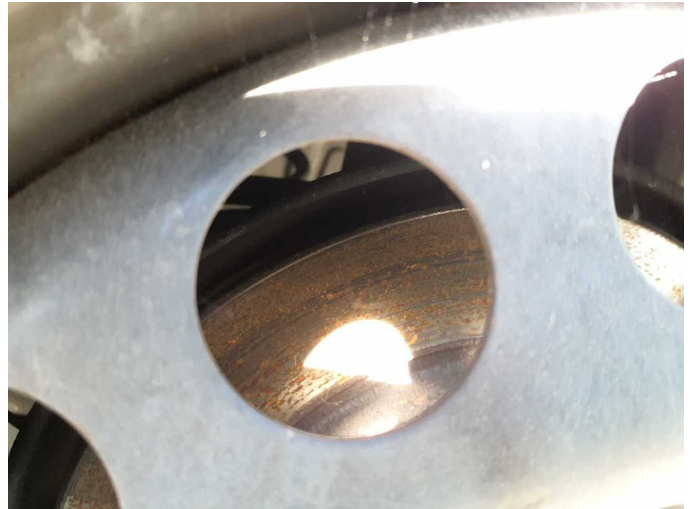
Wear and tear 3: Braking system: Brake discs and pads - rear - Corrosion - No deduction
