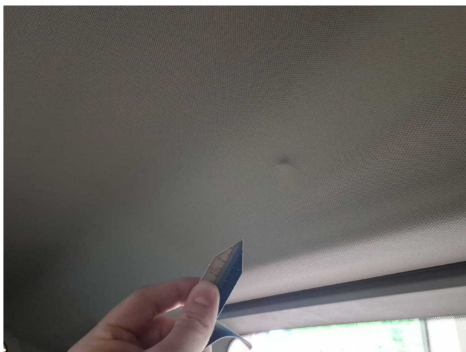
Wear and tear 4: Trim / covers: Roof lining - dent(s) - No deduction
