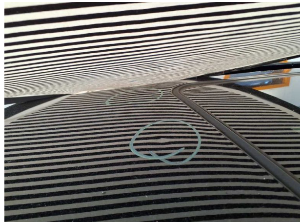
Damage #11: Roof: Roof - dent(s) - Smooth repair work
