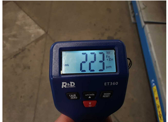
Roof rail - right side: 223 µm
