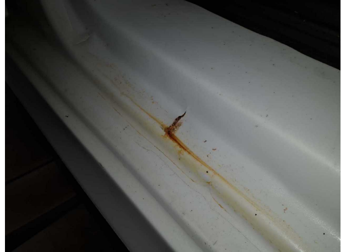
Damage 6: Sill - left side: Sill (Hinten) - Broken / torn - repair according to calculation
