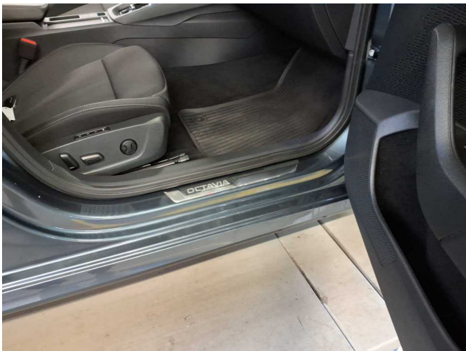
Damage 2: Sill - right side: Sill (Emblem, lack blättert ab) - Paint defect - Replace
