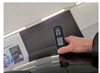
Paint thickness Roof
