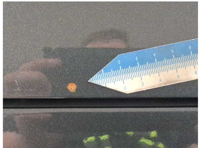
Damage 11: Bonnet: Bonnet - Corrosion - Paint
