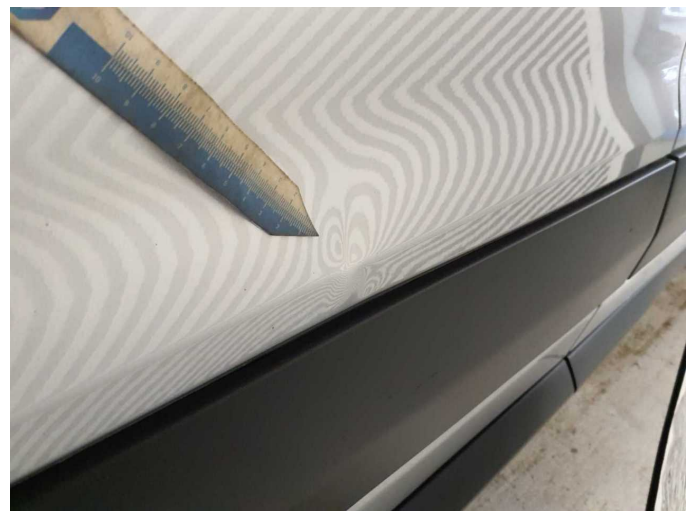
Damage 5: Sliding door, right: Sliding door with glass panel (Unterer Teil + Zierleiste erneuern) - dent(s) - Paint
