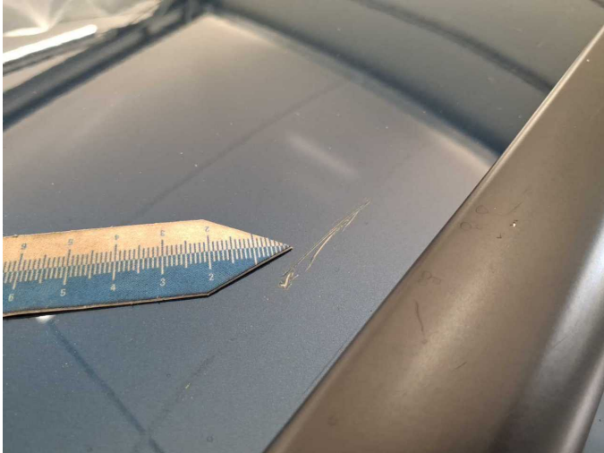
Damage 13: Roof: Roof (inkl. Railing) - Scratched - Paint
