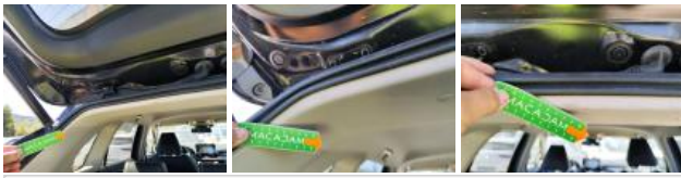
Inner door sill RR, Scratch(es), Acceptable
