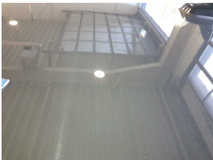
Damage 14: Roof: Roof - Scratch(es) - Paint
