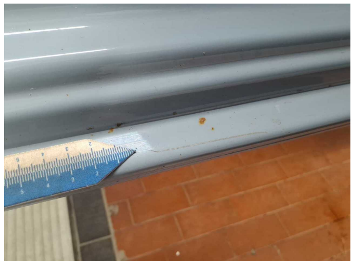
Damage 4: Sill - right side: Sill - Corrosion - Smart repair
