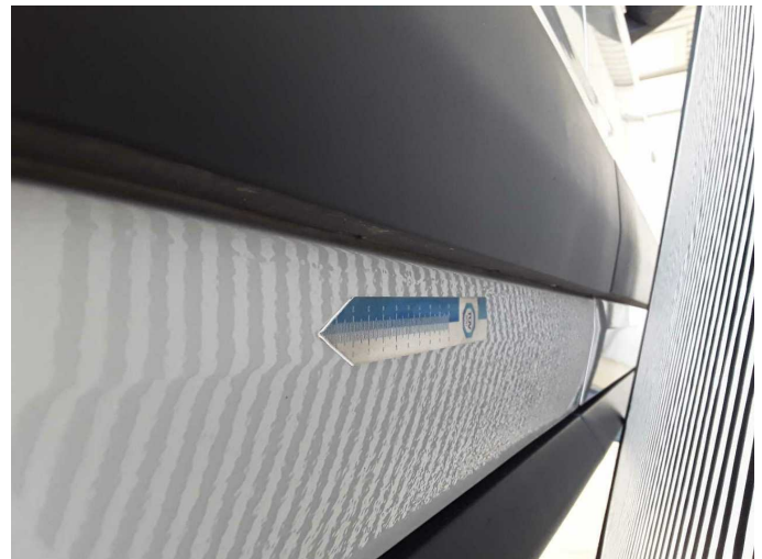
Damage 11: Sliding door, right: Sliding door (Läufer) - Unprofessionally repaired - Paint
