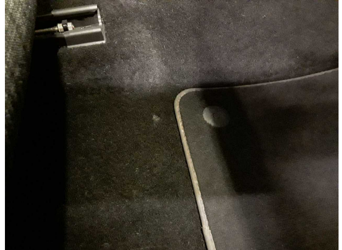
Damage 3: Trim / covers: Carpet - front right side - Burn hole (cigarettes) - Smart repair
