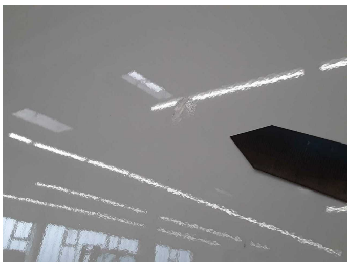
Damage 5: Sliding door, right: Sliding door (Orangenhaut, Schleifspuren) - Unprofessionally repaired - Paint
