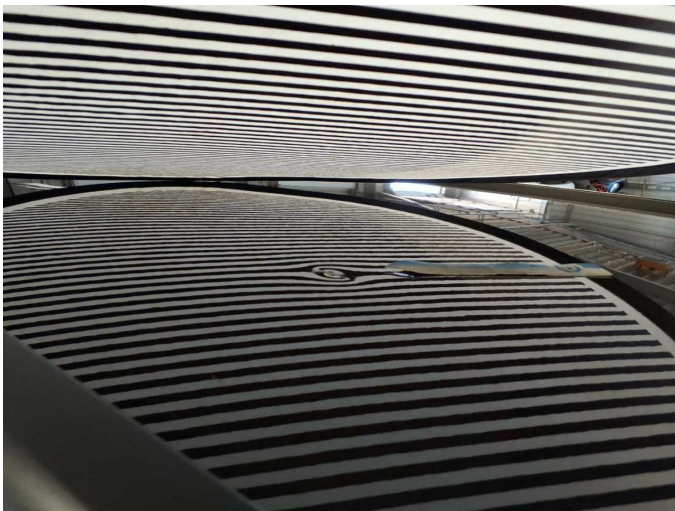
Damage 9: Roof: Roof - Dent / paintcoat damage - Repair and paint
