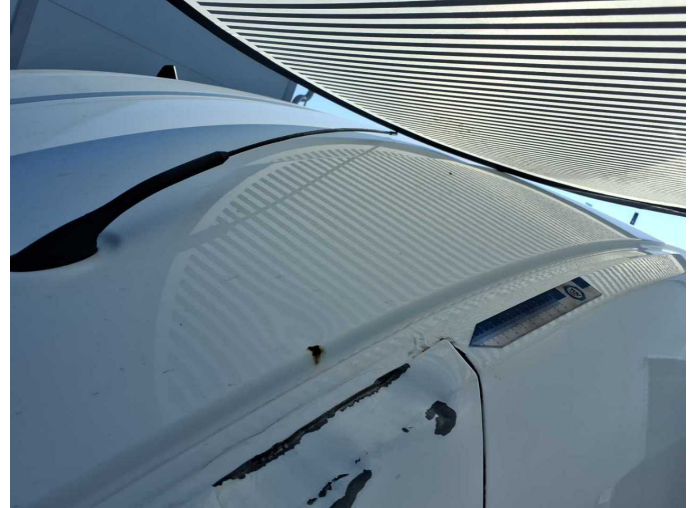
Accident 2: Roof, Front
