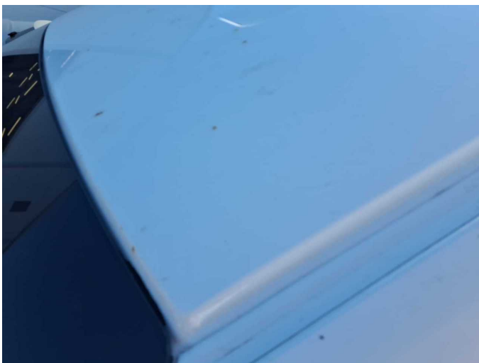
Accident 2: Roof, Front
