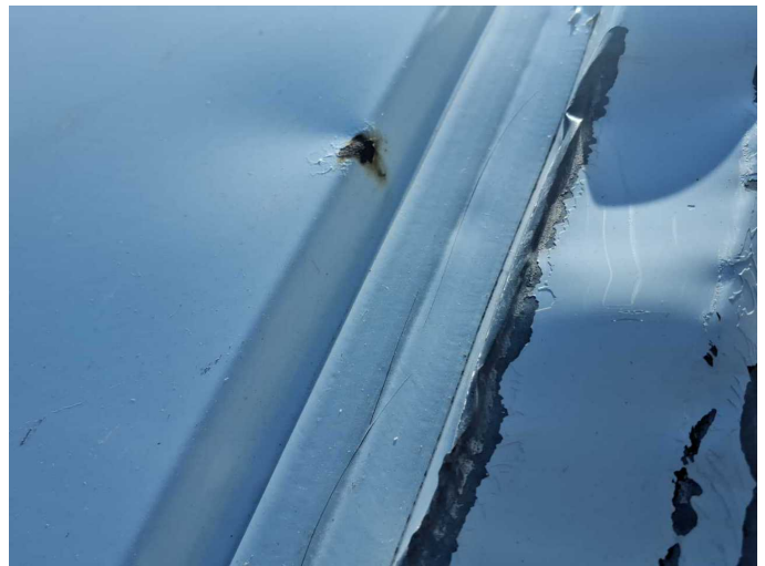
Accident 2: Roof, Front
