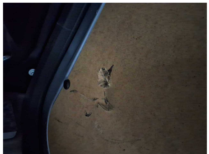
Damage 2: Sliding door, right: Trim plywood - lower - Broken / torn - Replace
