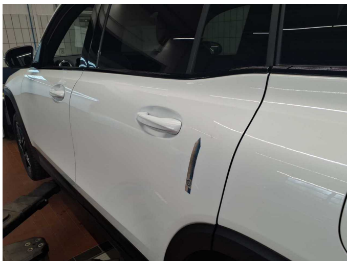
Damage 1: Body: Body (Flugrost) - Corrosion - Conditioning
