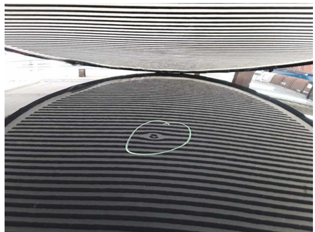
Damage #7: Roof: Roof - dent(s) - Smooth repair work
