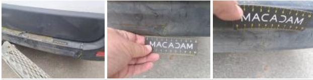
Rear bulkhead lining, Broken, Replace
