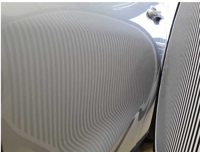
Damage 6: Door - rear left side: Door (Wellig) - Unprofessionally repaired - Repair and paint
