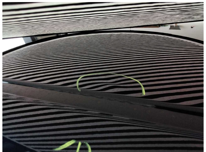
Damage 3: Roof: Roof - dent(s) - Smooth repair work
