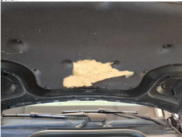
Damage #3: Bonnet: Insulation lining - Damage caused by martensite rodent - Replace
