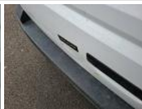
Supplementary brake light, Broken, Replace
