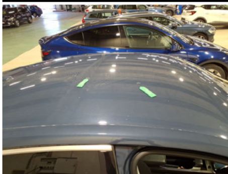
Roof / - / Paint etching
