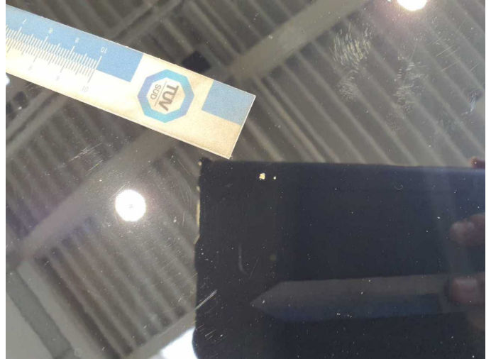
Damage 5: Roof: Roof - Stone chips - Paint
