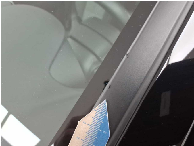
Damage 2: Roof: Cowl - left side - Broken / torn - Replace
