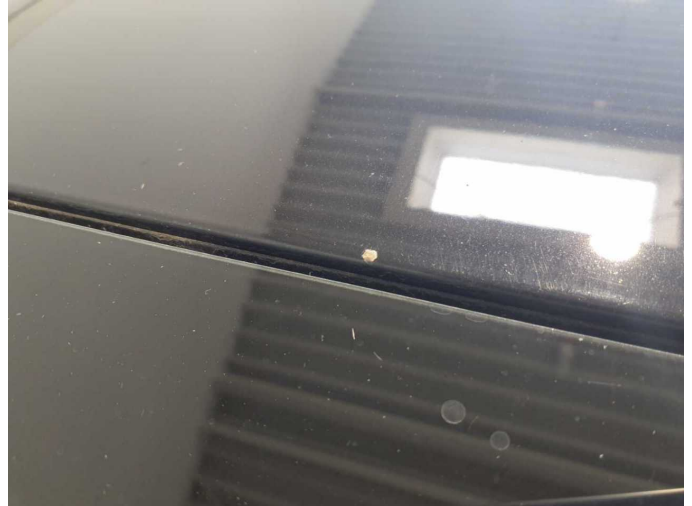
Damage 20: Roof: Roof - Corrosion - Repair and paint
