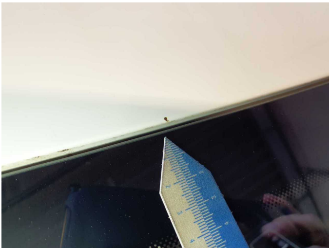
Damage 6: Roof: Roof - Corrosion - Smart repair
