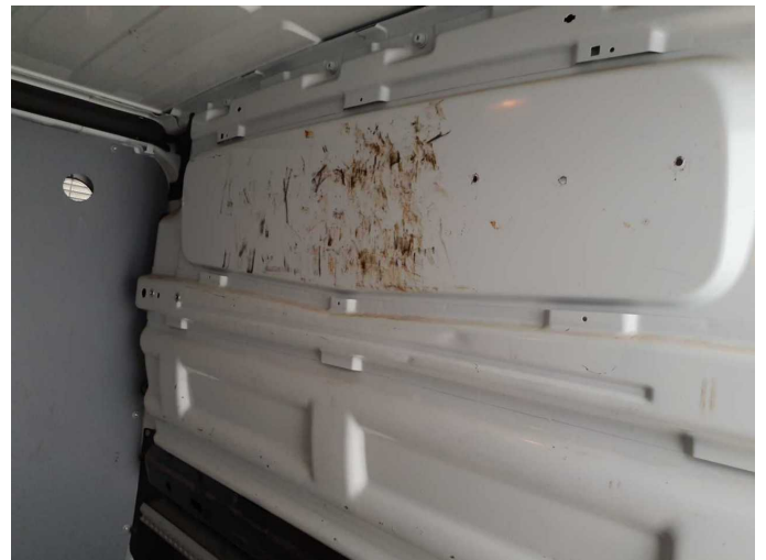
Damage 13: Body: Partition wall - Holes - Replace
