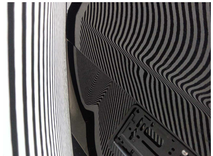
Damage 6: Boot lid / rear door: Boot lid - Dent / paintcoat damage - Repair and paint
