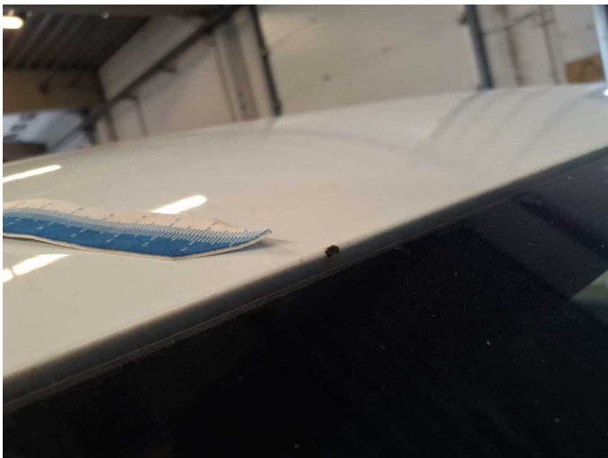
Damage 4: Roof: Roof - Stone chips - Paint
