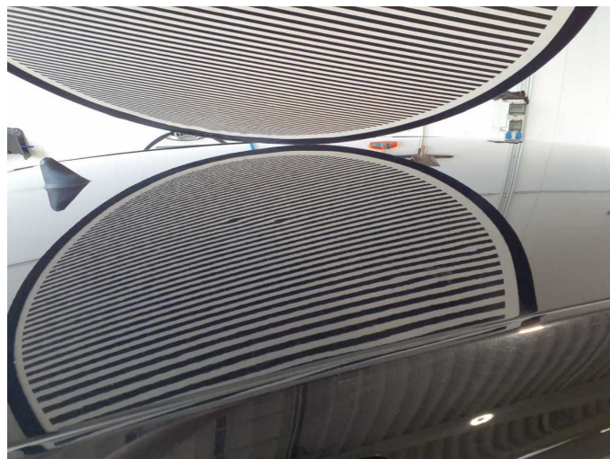
Damage 15: Roof: Roof (Korrosion) - Dent / paintcoat damage - Repair and paint
