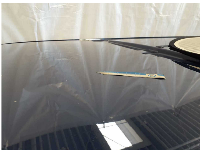
Damage 22: Roof: Roof - Dent / paintcoat damage - Repair and paint
