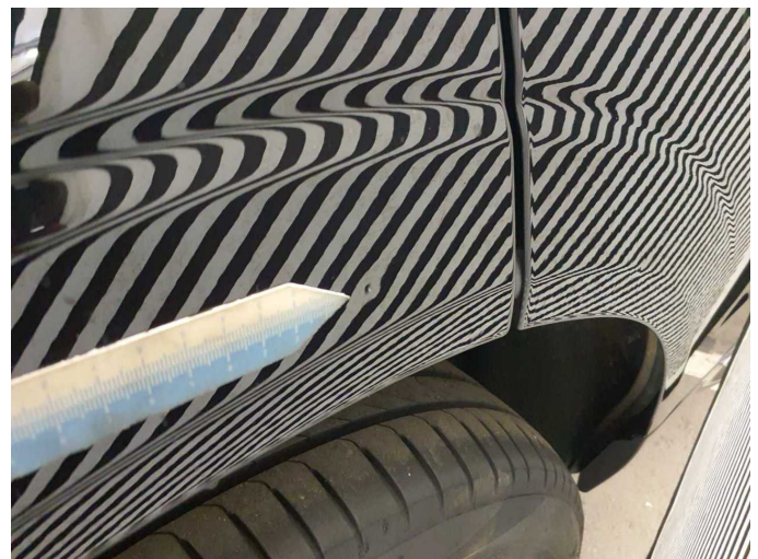
Wear and tear 5: Side panel - rear right side: Side panel - Dent / paintcoat damage - No deduction
