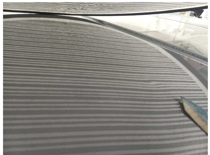
Damage 4: Roof: Roof - dent(s) - Smooth repair work
