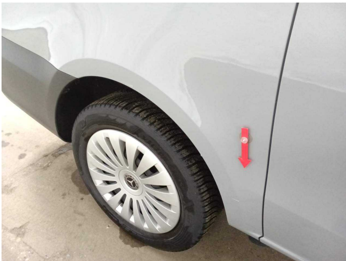
Damage 7: Side panel - rear right side: Elbow - Dent / paintcoat damage - Smart repair
