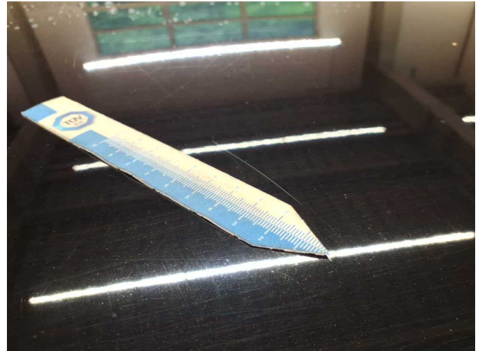
Damage 14: Roof: Roof - Scratch(es) - Paint
