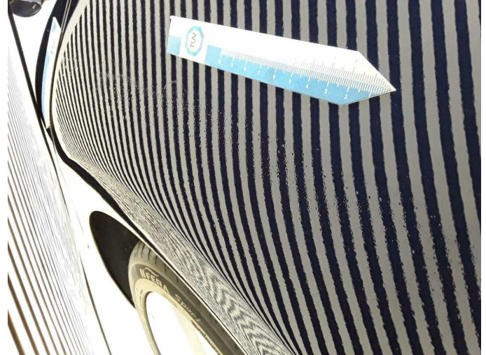
Damage 6: Side panel - rear left side: Side panel (Einschlüsse) - Unprofessionally repaired - Repair and paint
