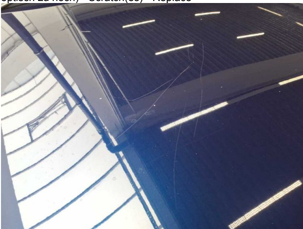
Damage #6: Roof: Roof - Scratch(es) - Repair and paint
